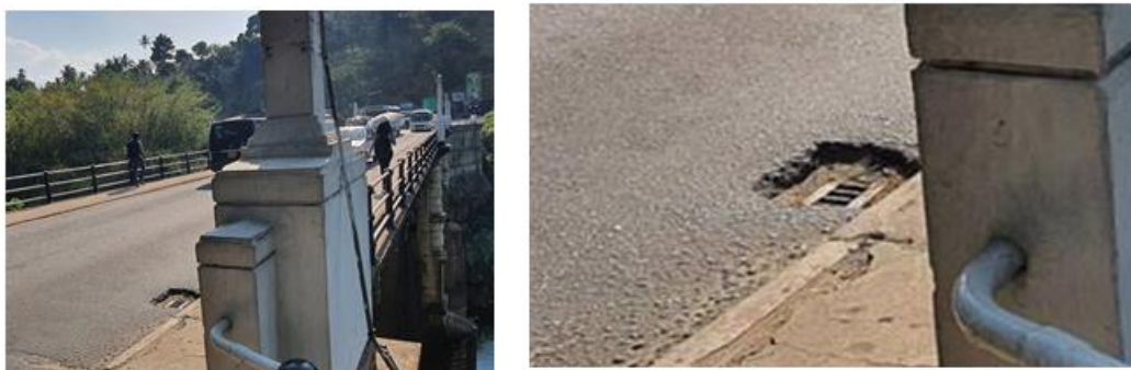
Figure 5.50 Drainage facility in the existing bridge
