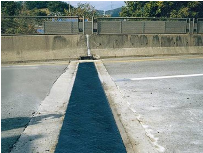
Figure 5.47 Asphaltic plug joint used in connection of bridges
