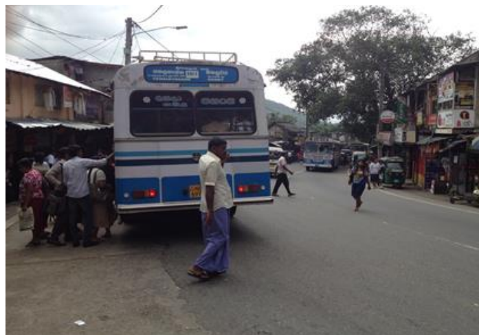
Figure 2.3 Improper design of bus-bays
