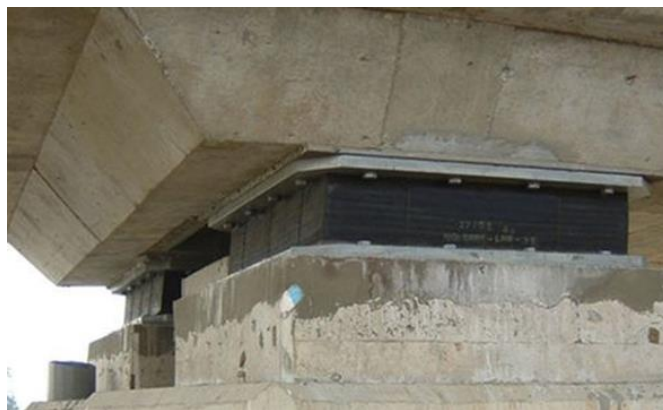
Figure 5.44 A typical bridge bearing
